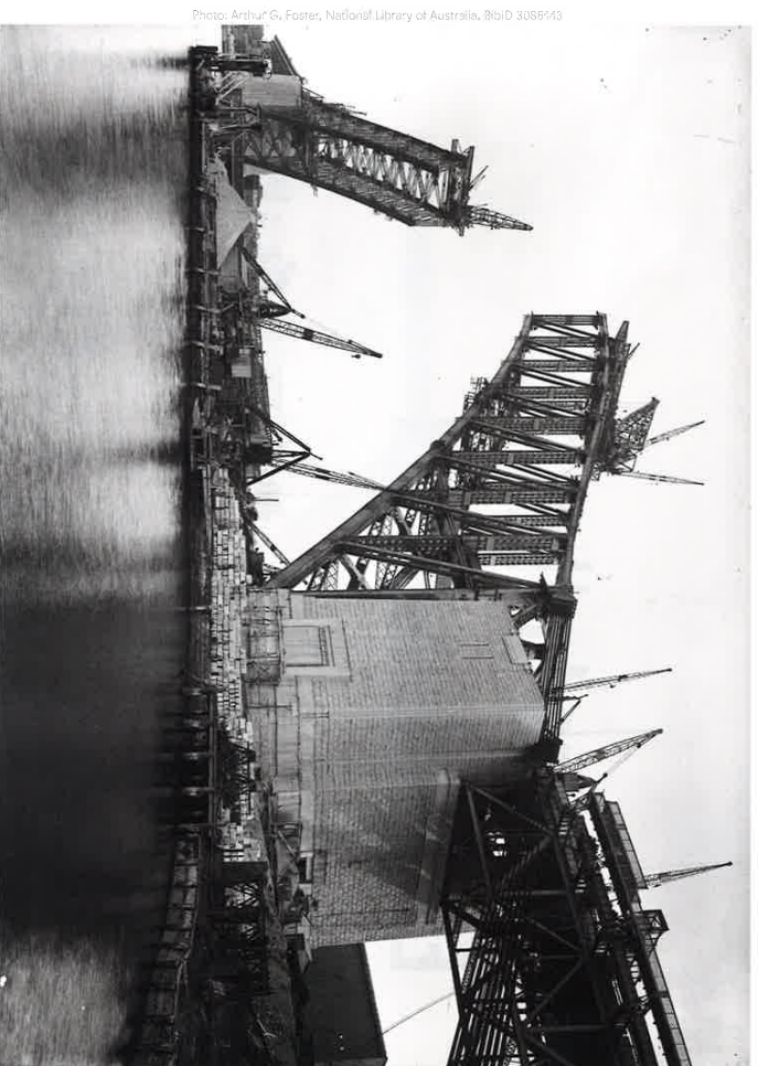
Construction of the Sydney Harbour Bridge (1923-32) with pylons of granite blocks sourced from the Moruya Quarry in Yuin Country
